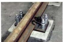
CRP on an underpoured socle
