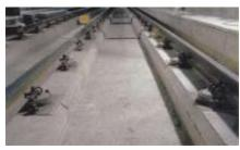
Cologne Egg, type CF1572 on concrete longitudinal plinths
